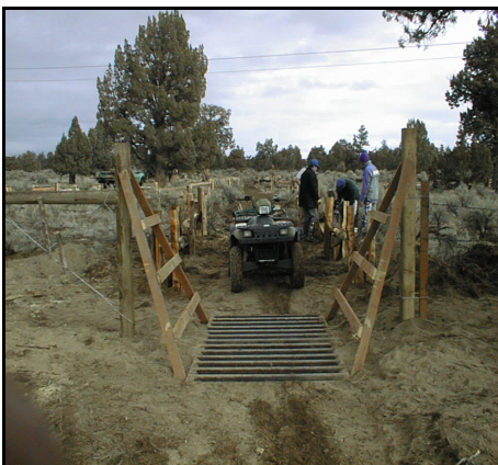
Members of Central Oregon Motorcycle and ATV Club installing a trail cattleguard and fencing at an OHV staging area.
